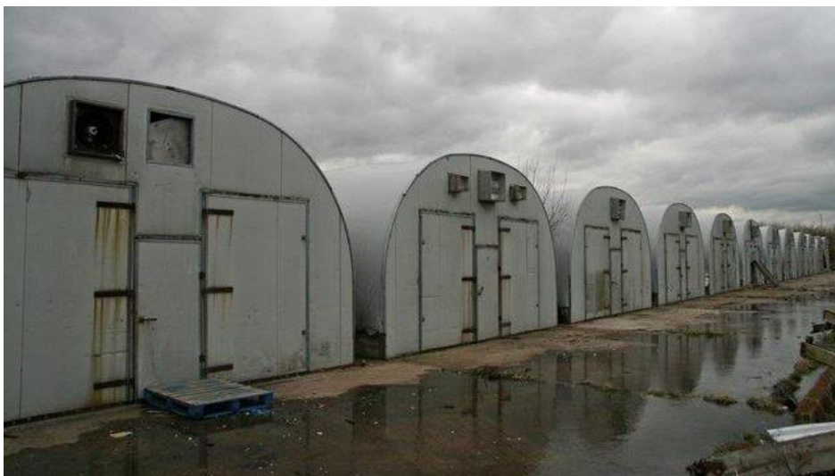
Mushroom sheds at the Gateforth site
